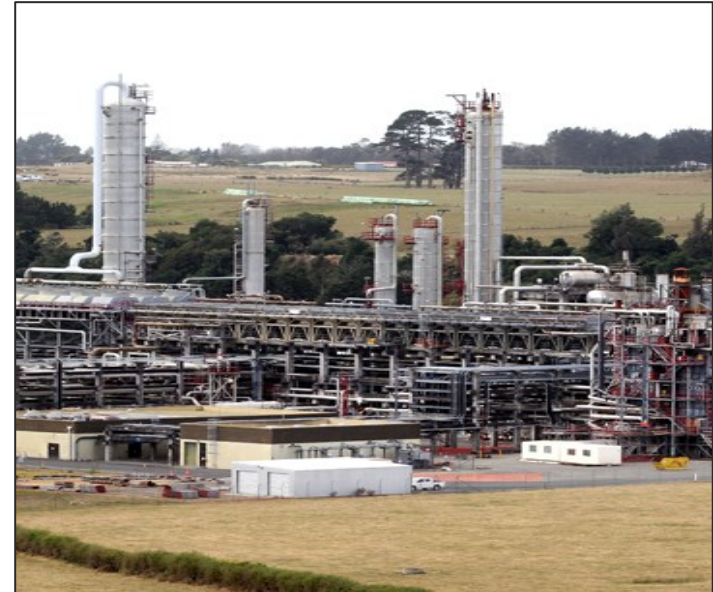
Waitara Valley Methanol Plant
